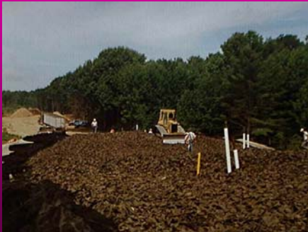
Overview of construction
