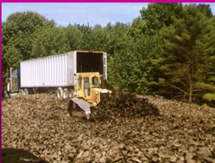
Spreading shreds with dozer
